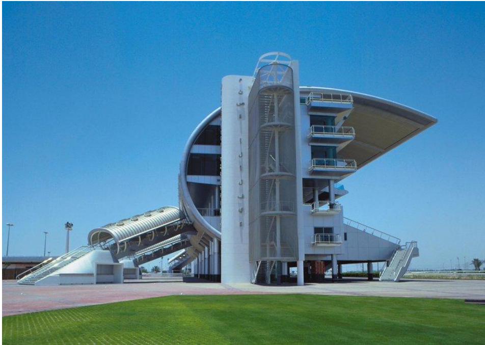
Φωτ 22. Grandstand, Dubai, UAE Kalzip.
