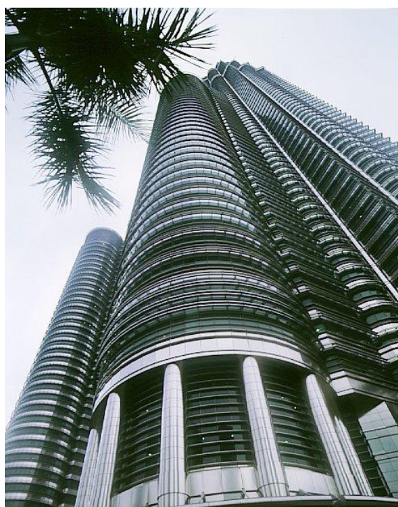
Φωτ 40. Petronas Twin Towers, Kuala Lumpur, Malaysia Alcoa Πηγή http://greenbuilding.world-aluminium.org/benefits/flexible/the-wave.html
