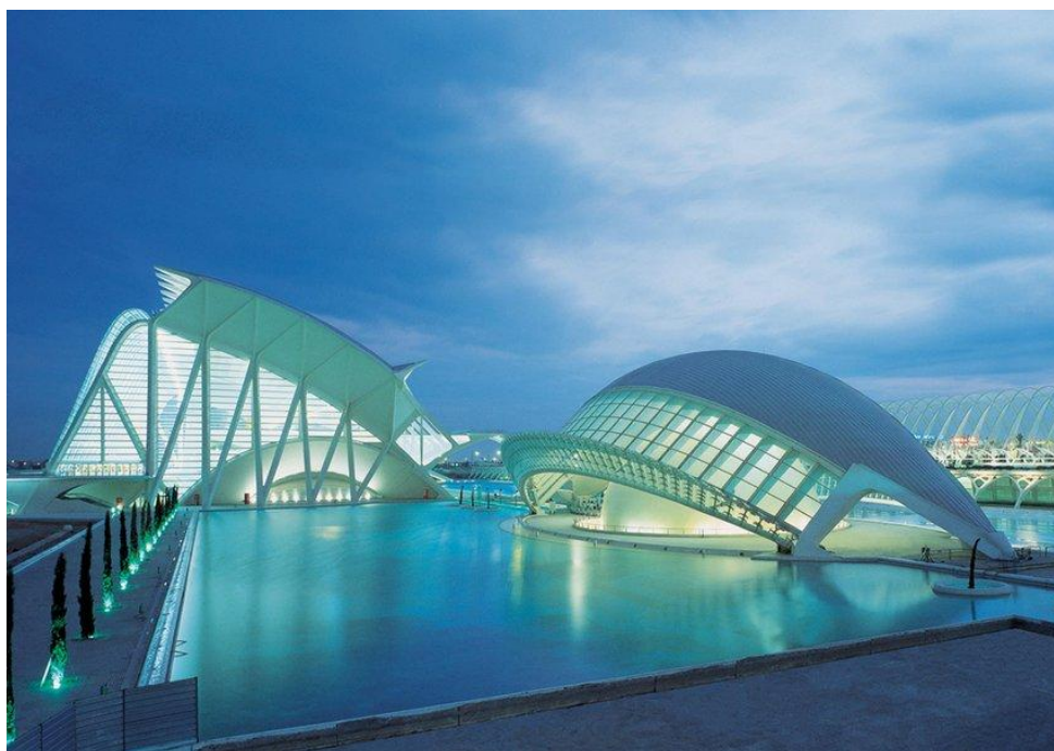
Φωτ 20. Science Museum, Valencia, Spain Kalzip.
