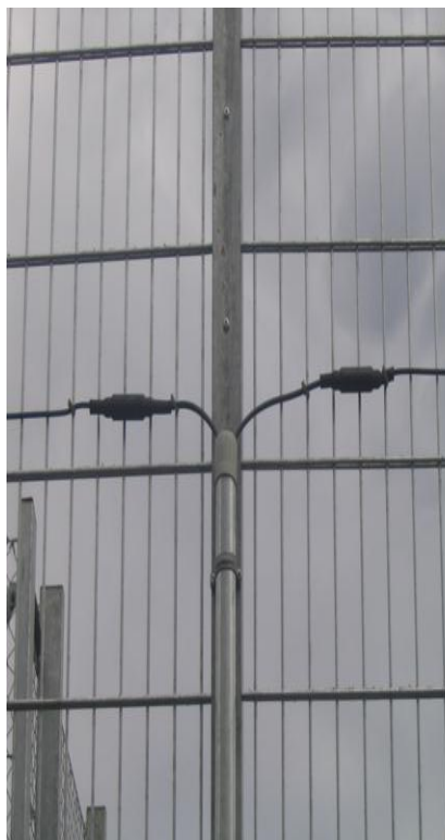
Figure 18. Cable Tie Placement - Gates & Maintenance Loops
