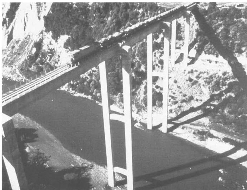
Fig. 3.11 South Rangitikei River Bridge.
