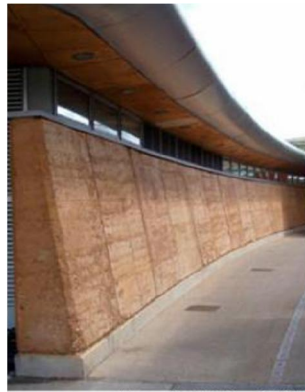
© Grimshaw architects; In Situ, Rammed Earth, 1999 Figure 1 Rammed earth wall construction at the Eden Project, Cornwall
