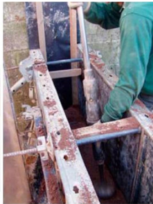
Figure 2 Construction of a rammed earth wall
